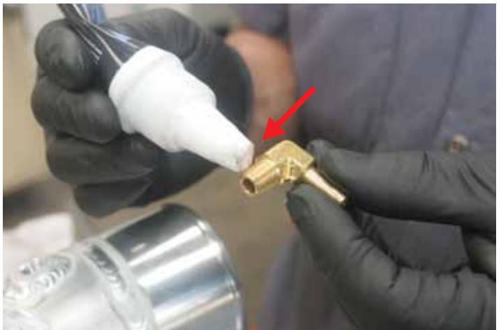
STEP 29 Install brass fitting using Teflon tape, fitting should face rearward, second port is for boost gauge.
